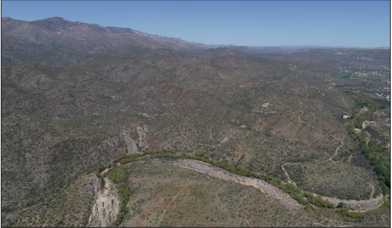
Figure 3. Aerial view of the project looking north.
